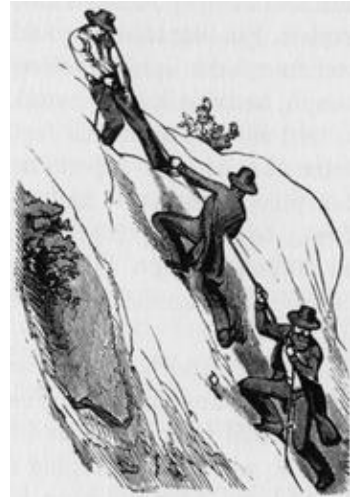
ASCENDING THE LOWER DOME.
