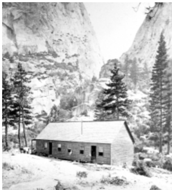
Snow's original "Alpine House" was a barebones structure with little charm.
