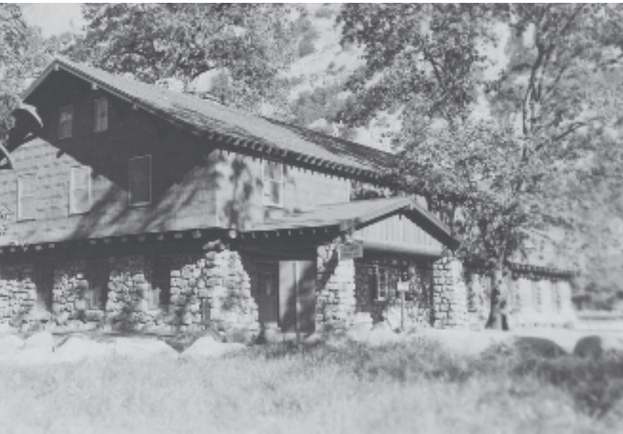
Yosemite Administration Building, seen in 1926.
