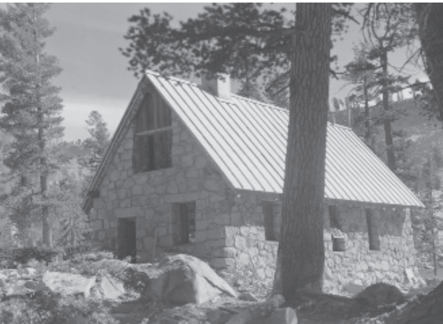
The stone work of the Ostrander Ski Hut (1940) reflects its rugged surroundings.
