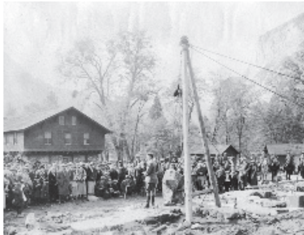
The construction of the Museum. Ranger Ansel Hall, the impetus behind the Museum, stands beside the cornerstone; the Administration Building can be seen in the background.
