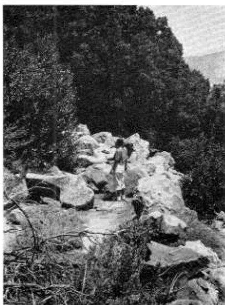
One of the many rock slides now obstructing the old Big Oak Flat Road.
