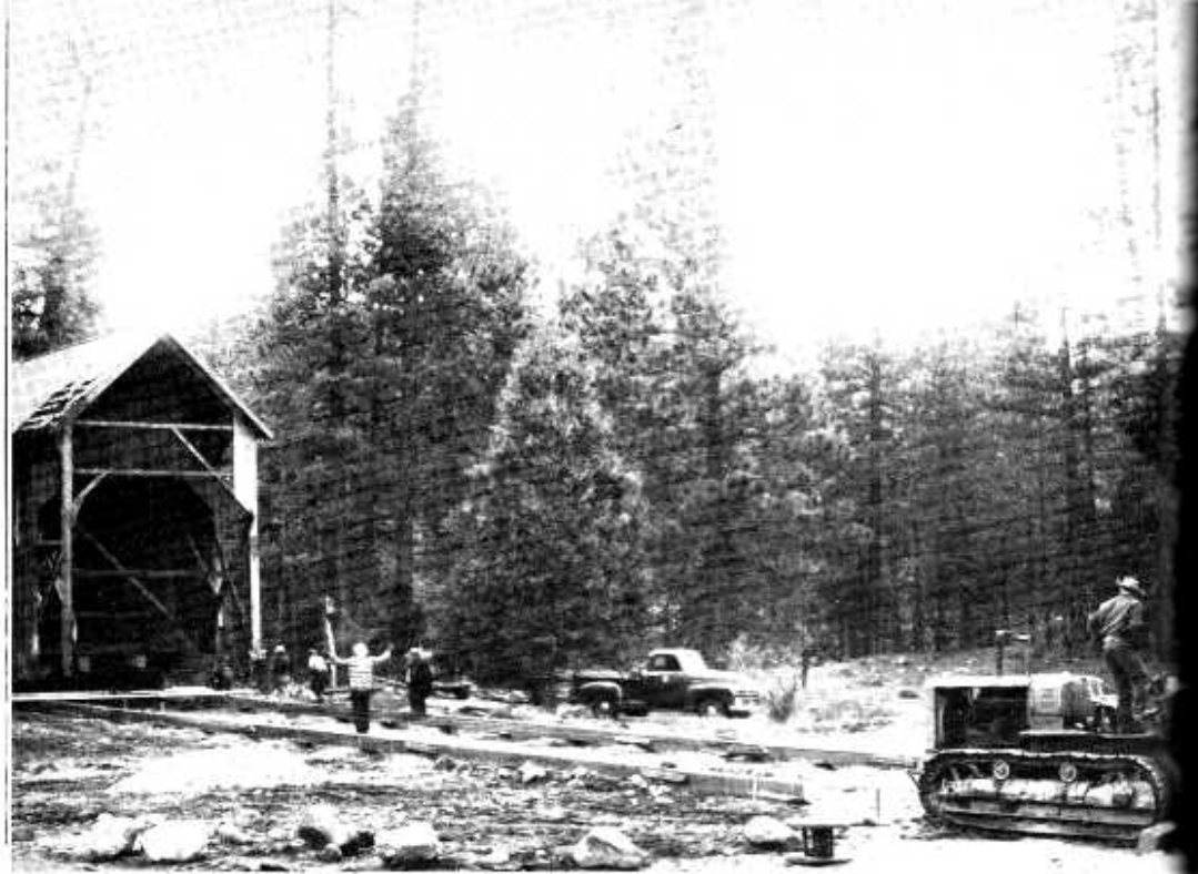
The bridge moved smoothly ashore.
