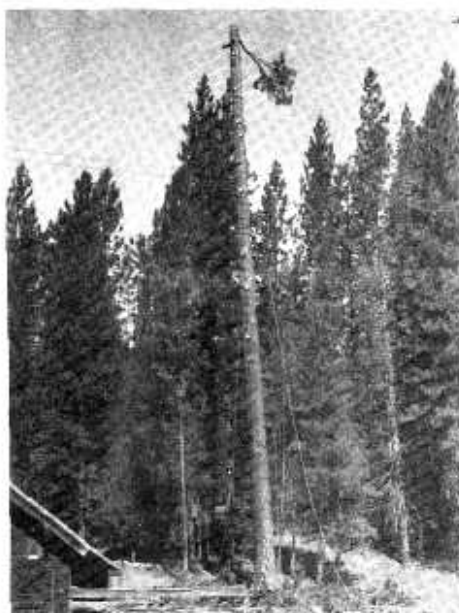
Topping tree for bridge supports.
