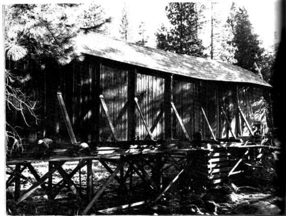
After the flood of 1955 cribbing saved the bridge.
