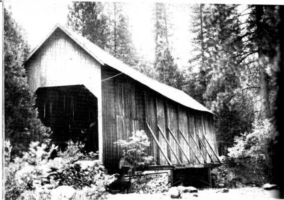
In 1955 the bridge was beginning to sag.
