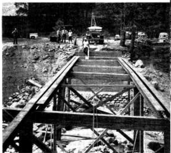
A "track" was made to pull the bridge back into place.
