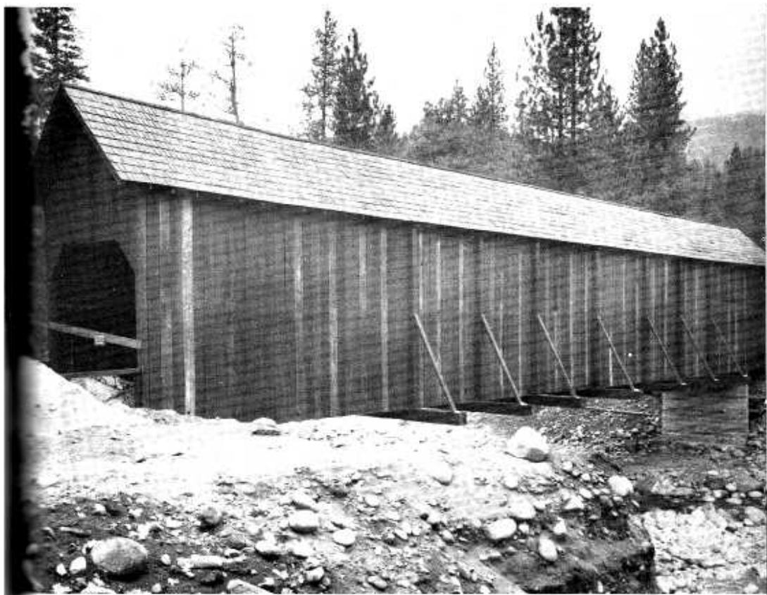
The bridge as it appears today. Only rock work and fill remain to complete the job.
