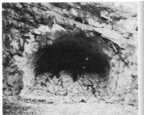
Starting the Wawona Tunnel, 1931.
