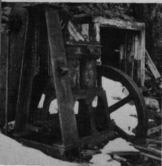
Machinery Hauled Over the Snow in 1882; Great Sierra Tunnel at Right.
