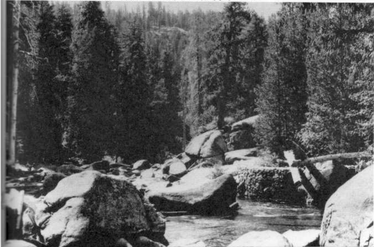
6. Looking downstream toward the 1956 diversion wall at the top of Liberty Cap gully in 1999.
