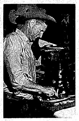
Using a skiving tool to trim leather to proper thickness for stitching or riveting.
